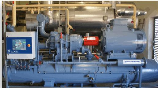
Our open-architecture retrofit screw compressor control package is the solution you're looking for. The eLOGIC controller is based on our Signal Server Technology design platform and over 40 years of experience in the design, development, and implementation of scalable refrigeration control systems.
